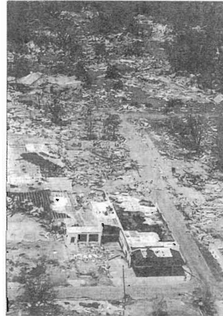
MARKET STREET LOOKING NORTH AFTER KATRINA WE CANNOT CONTROL FLOODS OR HURRICANES, BUT WE CAN CONTROL FLOOD/HURRICANE DAMAGE.
