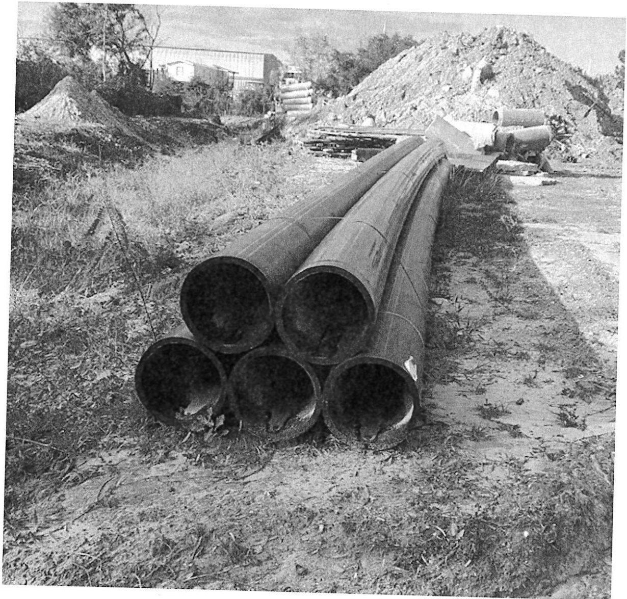
1257 North St. HDPE Stored Materials
