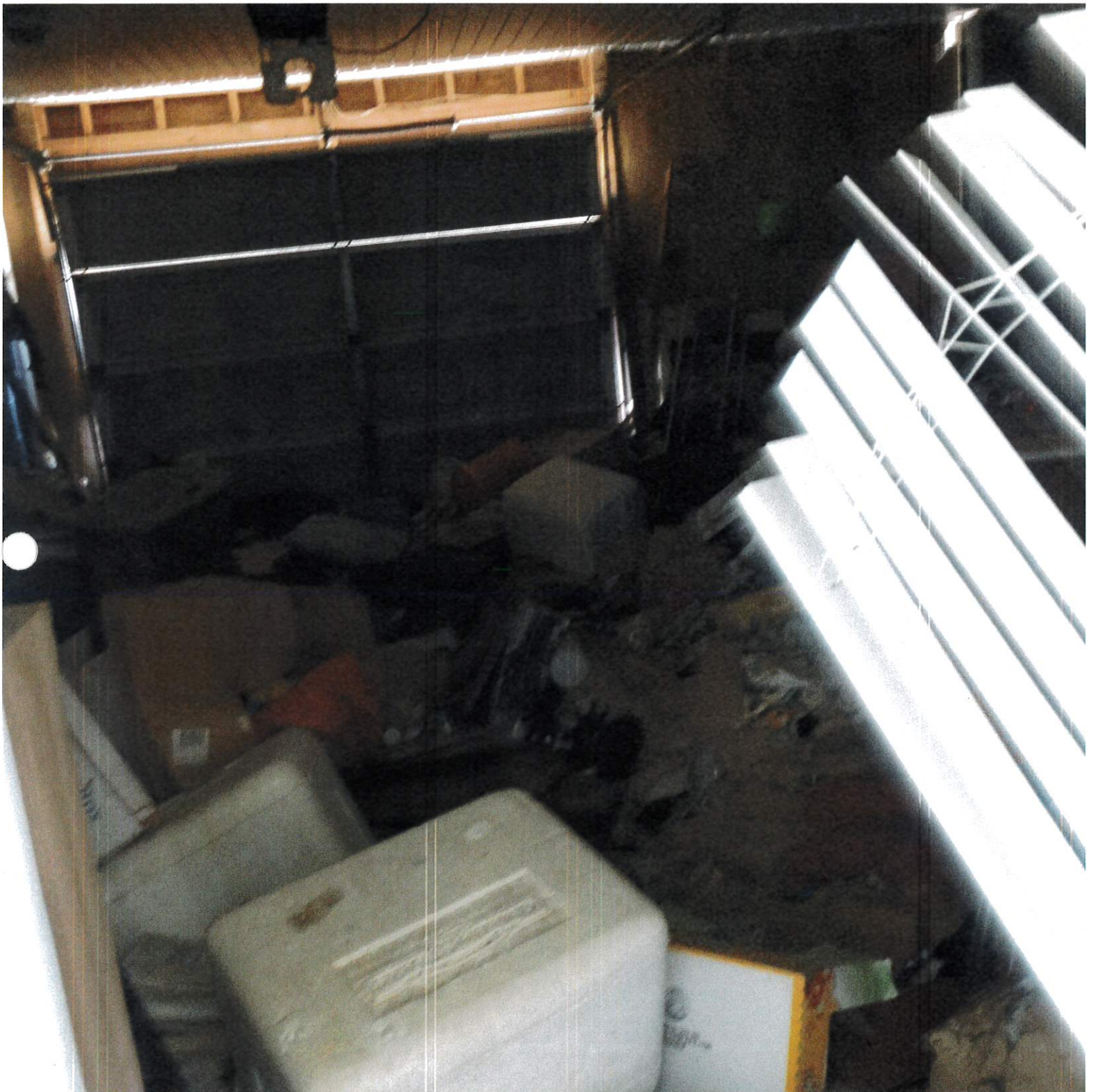
INSIDE GARAGE, WASTE PILED WAIST DEEP
